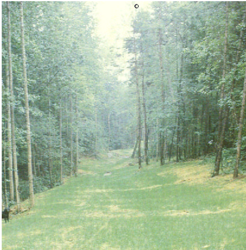
Right-of-way diversions (water bars) prevent erosion from long narrow slopes.
