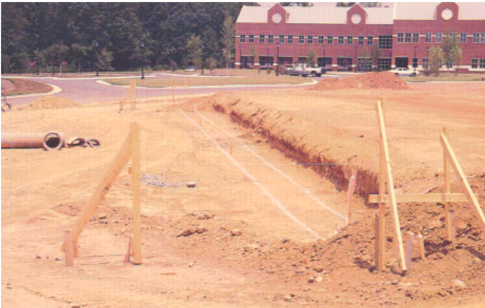
Land grading shapes the surface to a specific line and grade.
