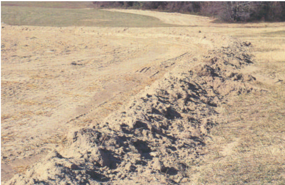
Temporary diversion across a slope helps prevent sheet and rill erosion.
